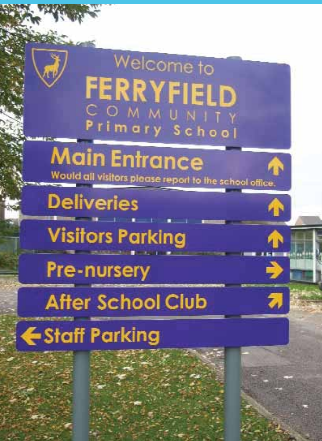
This large multi-panel sign has three posts to meet wind loading requirements
